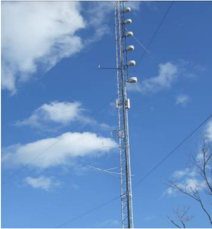
Figure 2. Photo of Lutsen communication tower showing anemometer extending laterally from tower.
